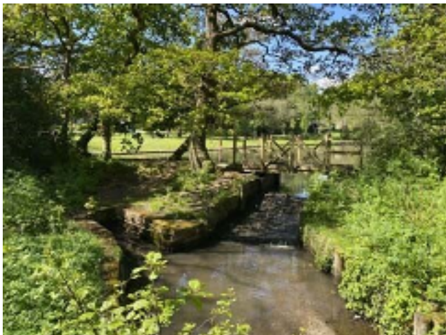
Existing footbridge (image taken from Fernhill Lane)
