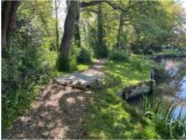
Existing raised service structure
