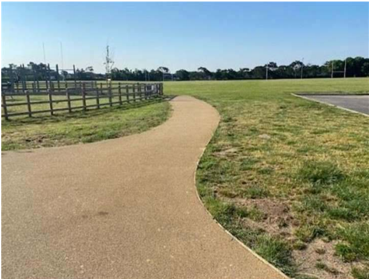
An example of the planned buff tarmac footpath, at Ashley recreation ground
